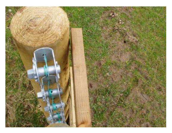
Note rails not nailed to strainer, so both sections of fence are completely separate.
