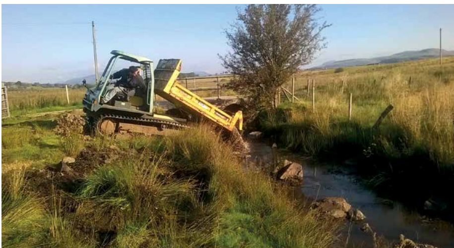
Figure 4. Clean gravel being seeded into the Afon Eden SAC. © Natural Resources Wales.
